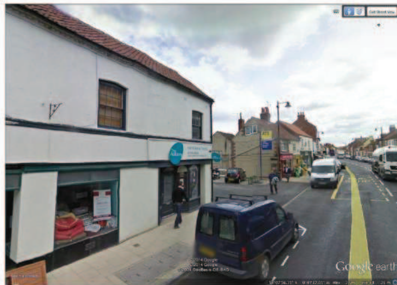
VIEW OF THE SITE ENTRANCE LOOKING EAST ALONG COMMERCIAL STREET
